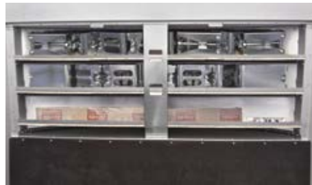
... or in the bulkhead.
